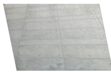
Ceiling & Wall Plaster
