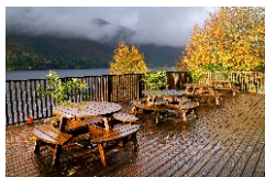
Exterior Wood Surfaces
